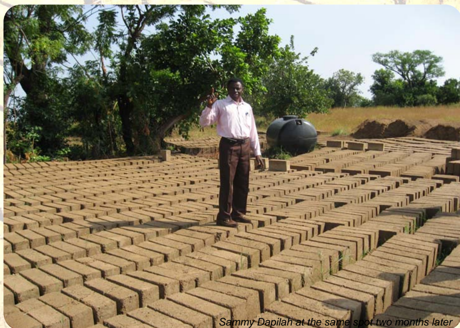
Construction of breeze blocks
