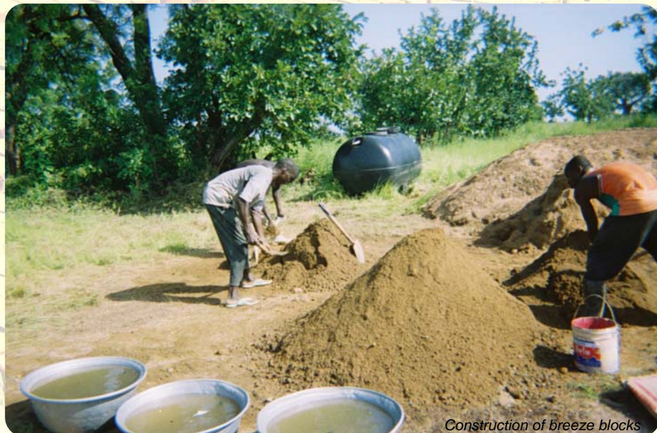
Construction of breeze blocks
