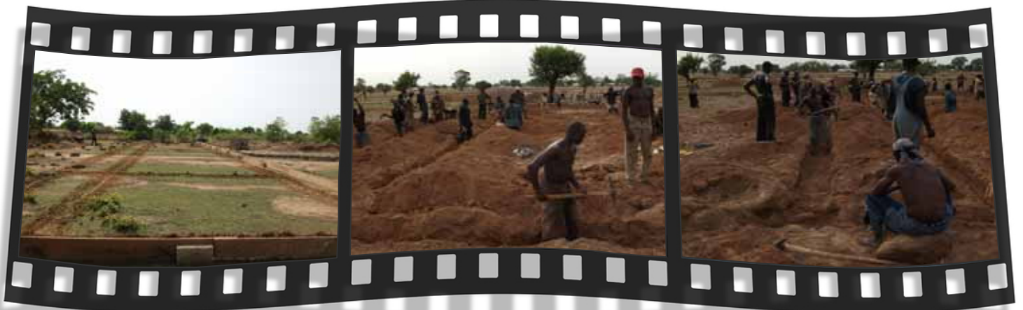
8. Digging foundations: the foundations are dug and the shape of the schools becomes clearer
