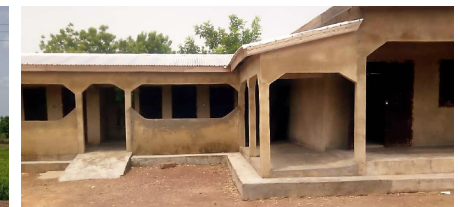
Significant building work at Danko Buree
