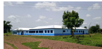
Painting completed at Baapari Primary School
